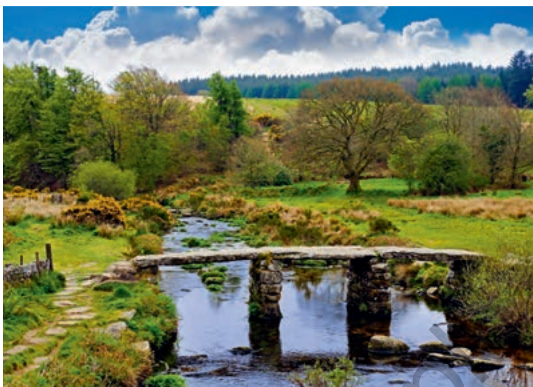
Clapper Bridge, Postbridge, Yelverton, Devon
